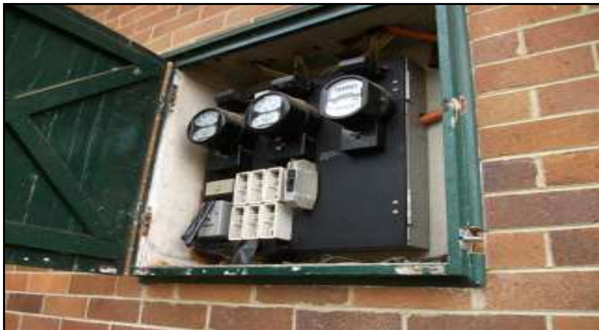
Figure 17 - Electrical Backing Board & Cement Lined Electrical Cabinet
