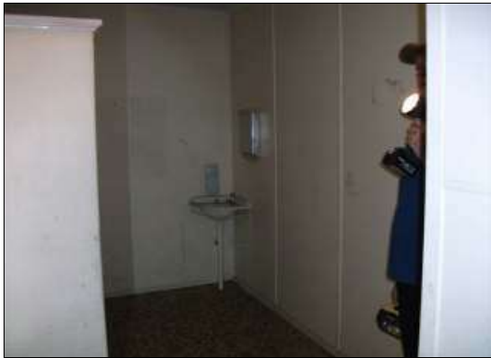
Figure 13 - Mens & Ladies Toilets - Fibre Cement Wall & Ceiling Panels
