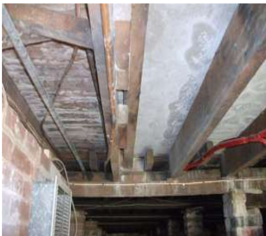
Figure 16 - Fibre Cement Used As Packing on Piers
