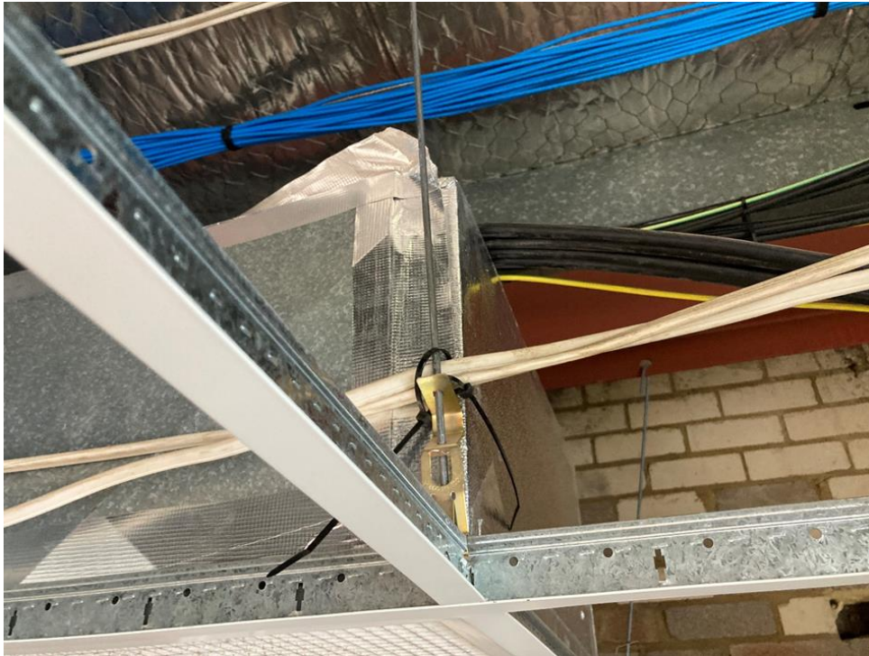
Electrical Sub Mains Cabling (Black Cables) laying on HVAC Ducting. Non-compliant with Australian Standard - AS3000
