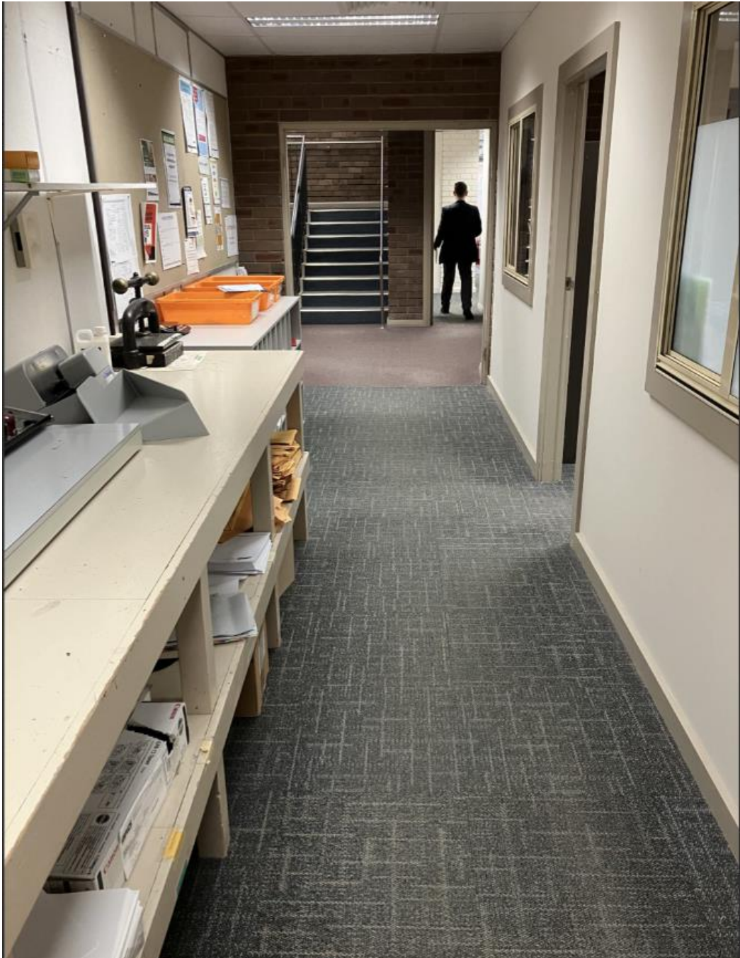
Minimal Storage - leading to items being placed in corridors and path of travel for fire egress
