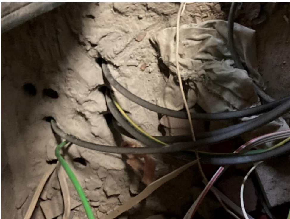
Electrical Sub Mains Cabling (Black Cables) laying on HVAC Ducting. Non-compliant with Australian Standard - AS3000
