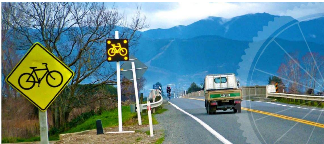
Figure 5.18: Bicycle Activated Warning Sign - Waimea River Bridge, Appleby (Tasman District Council)
