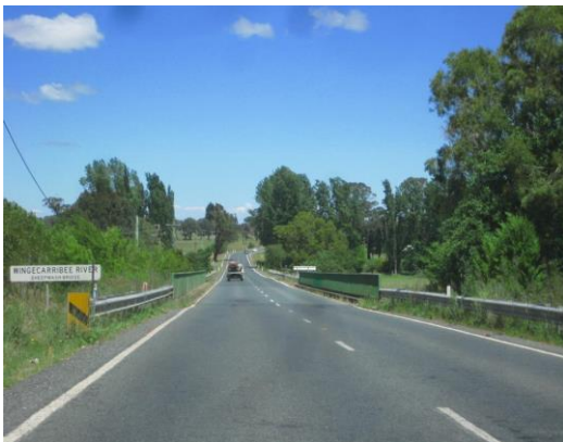
Figure 2.4: Sheepwash Bridge, Sheepwash Road, Glenquarry
