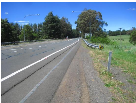
Figure 2.6: Illawarra Highway at Sheepwash Road, Avoca
