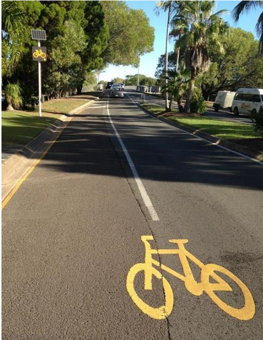
Figure 5.14: Bicycle activated warning sign – Noosa Parade, Noosa, Queensland
