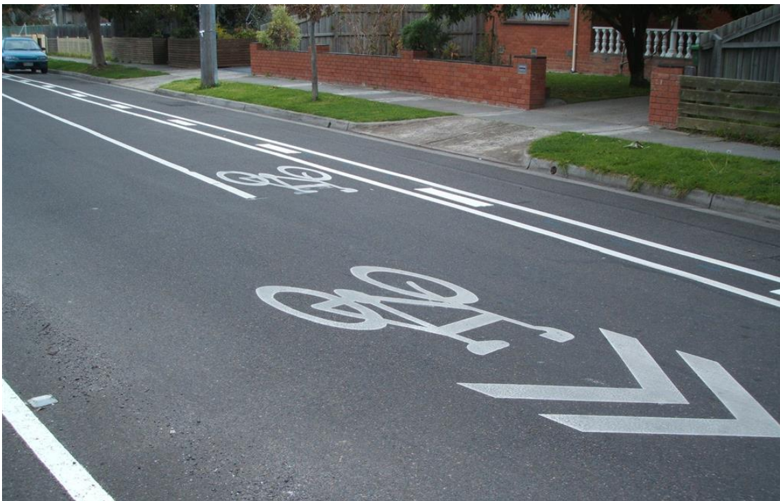
Figure 5.21: Sharrow Road Markings – Raglan Street, Preston, Victoria
