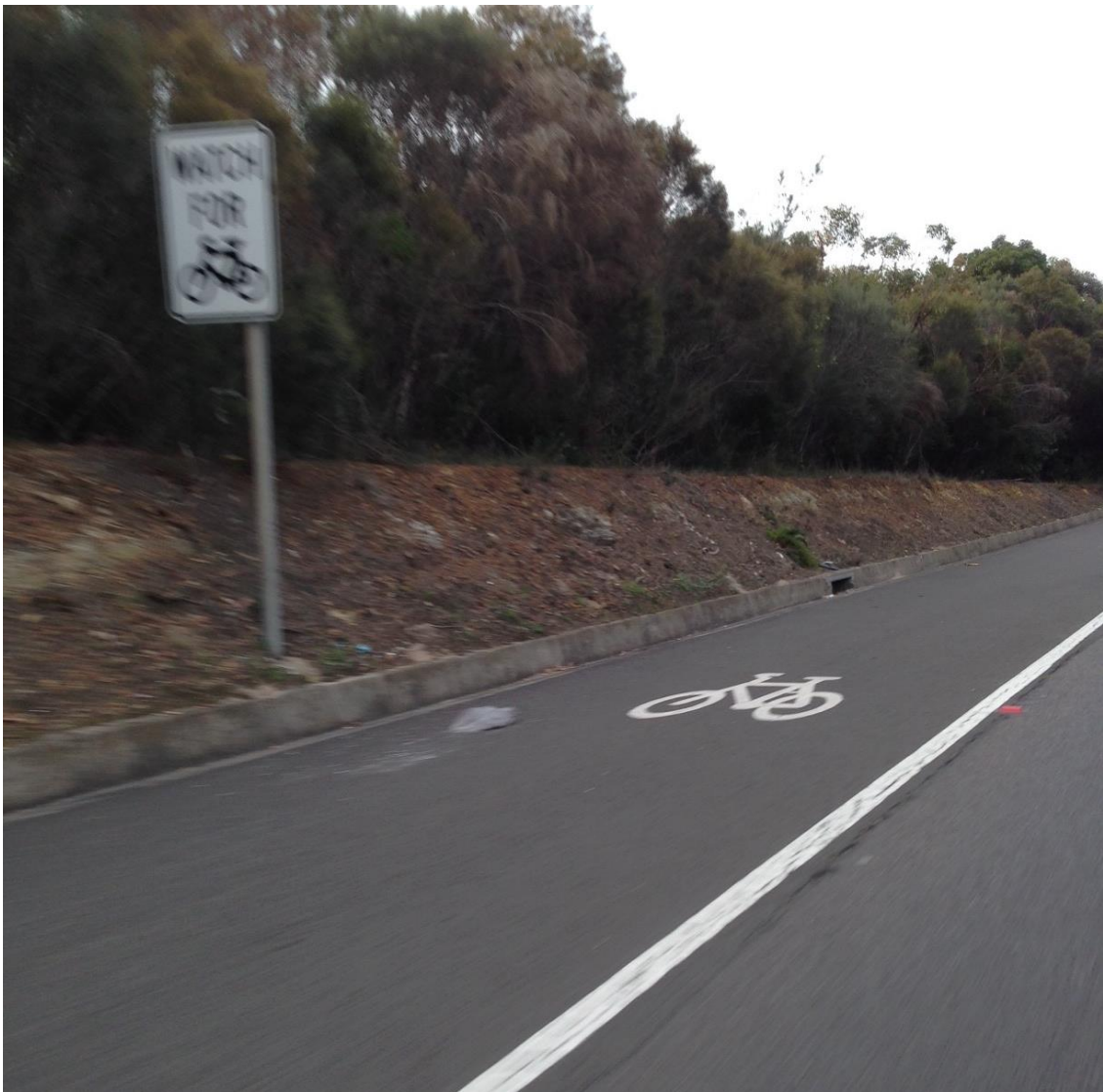
Figure 5.3: Typical motorway sealed shoulder treatment (Princes Motorway)
