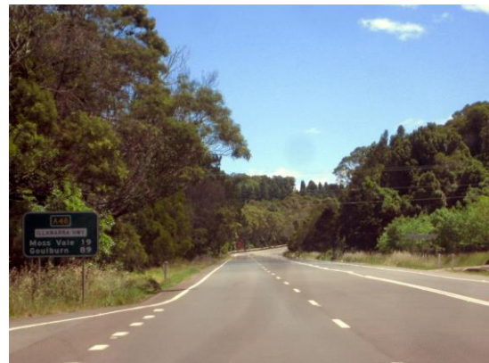
Figure 2.5: Illawarra Highway, Burrawang
