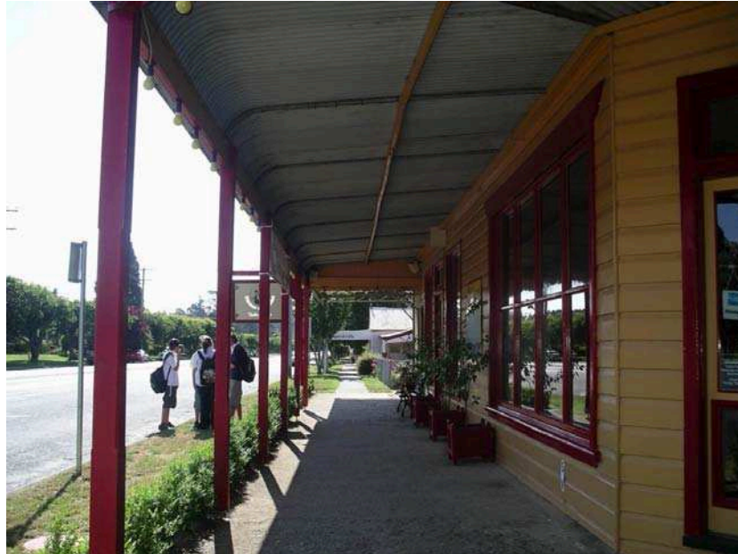
Figure 13: Veranda over footpath outside Waters Shop, Hoddle St
