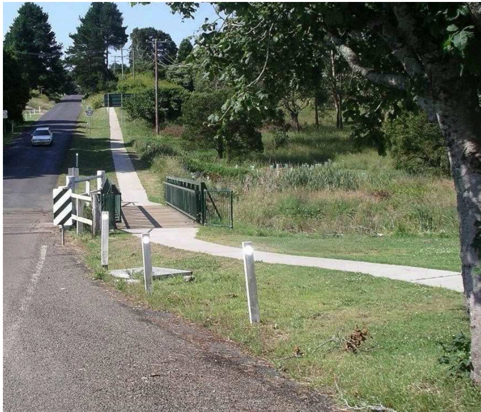
Figure 12: Caalong Street path showing footbridge
