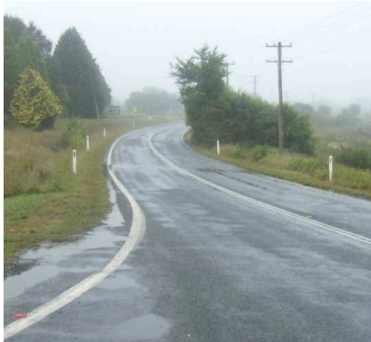
Figure 10: Illawarra Highway, east from East Street
