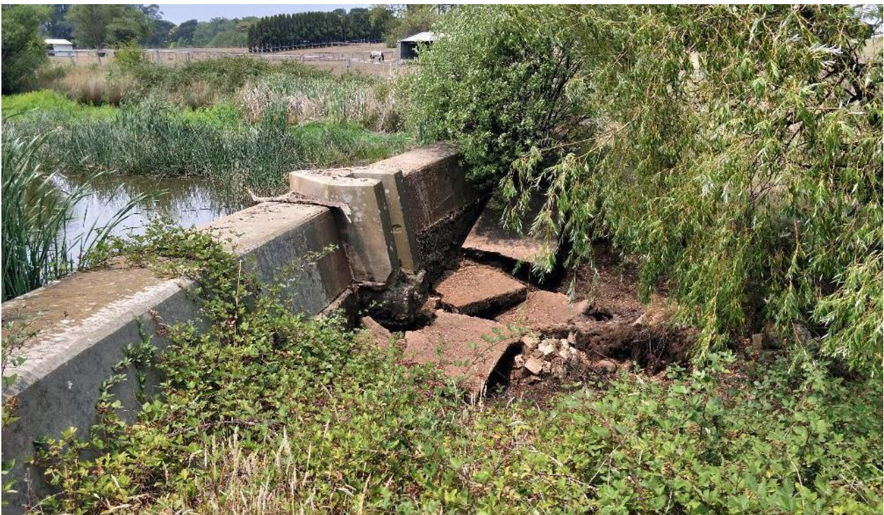
Figure 6-2 Existing weir along Mittagong Creek
