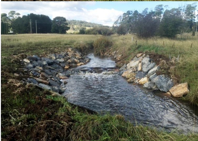
Figure 10 Rock ramp, one of three in-stream structures constructed in 2015.
