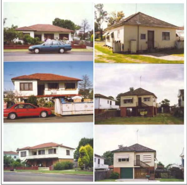
Plate 47 Examples of houses before (top image), during (middle image) and after (bottom image) house raising (photos courtesy of Fairfield City Council)
