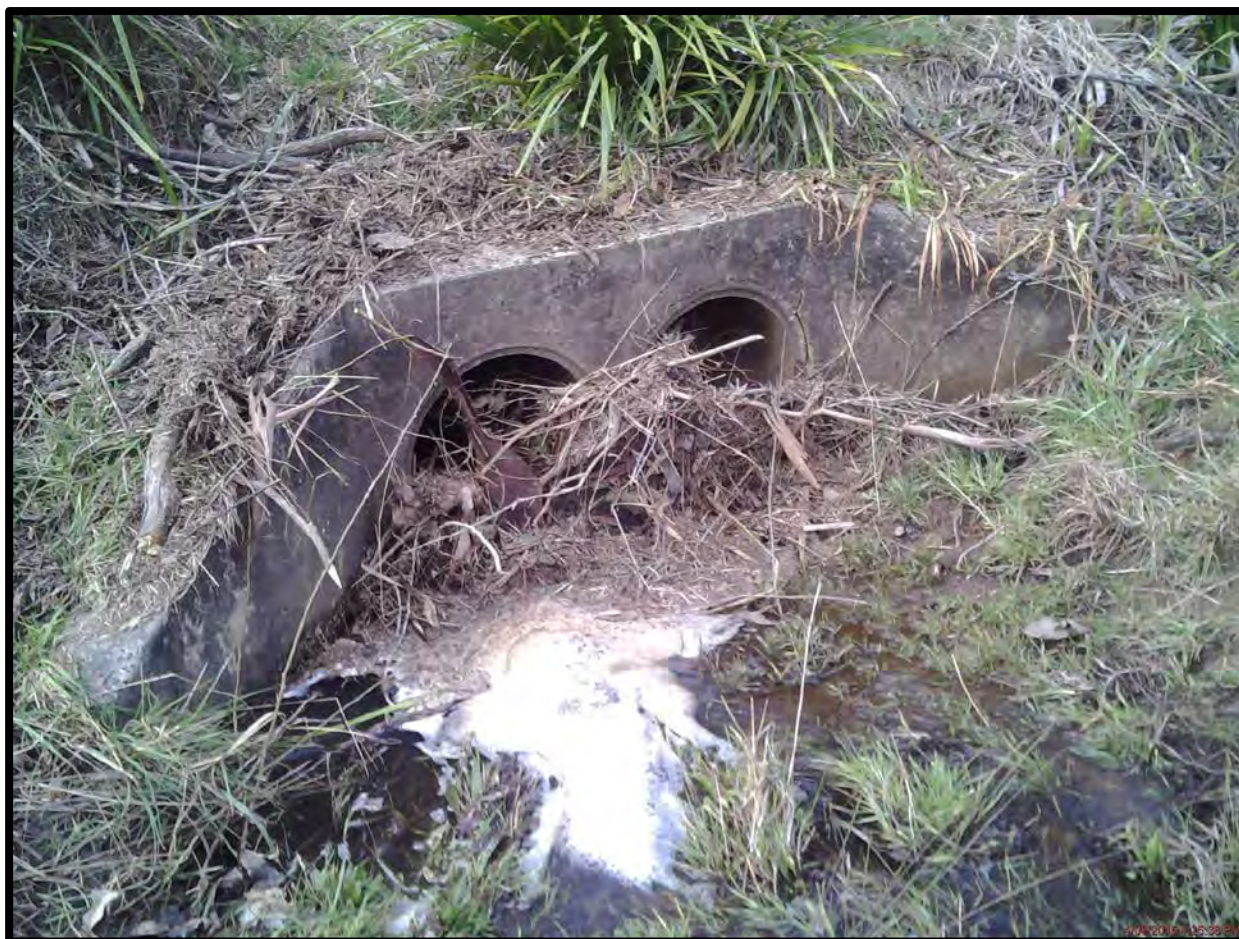
Plate 11 Example of vegetation and silt partially blocking culvert at rear of property at 14 Evans Street, Mittagong.
