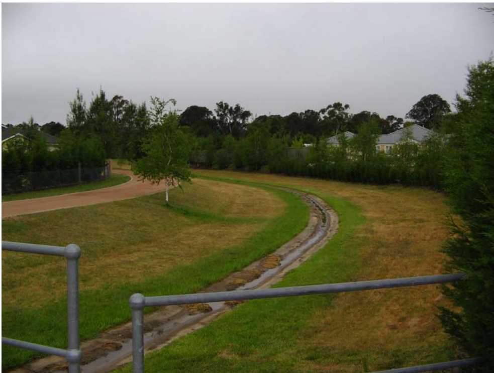
Lined invert to channel – near Stratford Way
