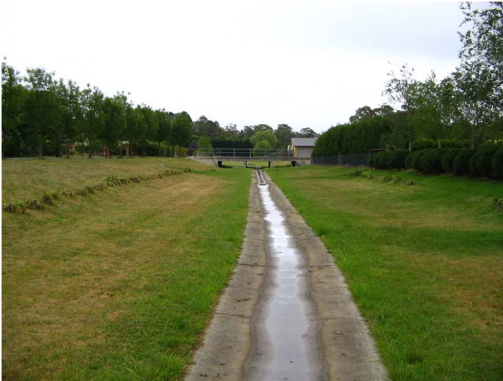
Lined invert to channel – near Stratford Way
