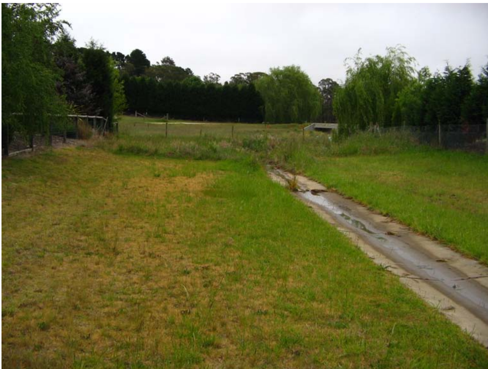
End of lined invert to channel – near Stratford Way
