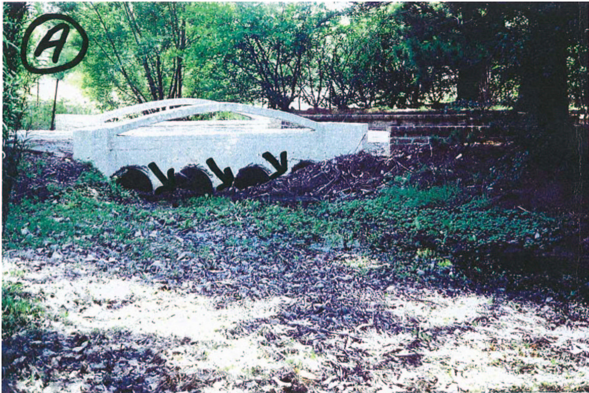
Driveway culvert at property on Holly Road – noting deposited debris at inlet
