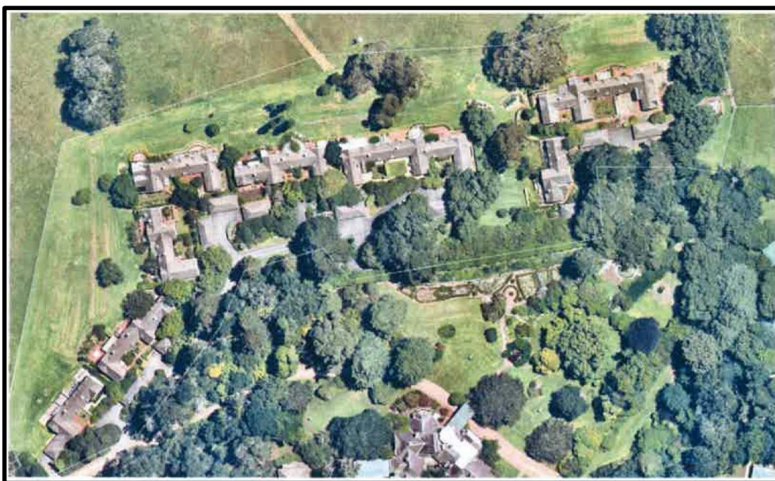
Figure 4: Aerial Photo of Village 1 (Attachment 4 (Source: Near Map))
