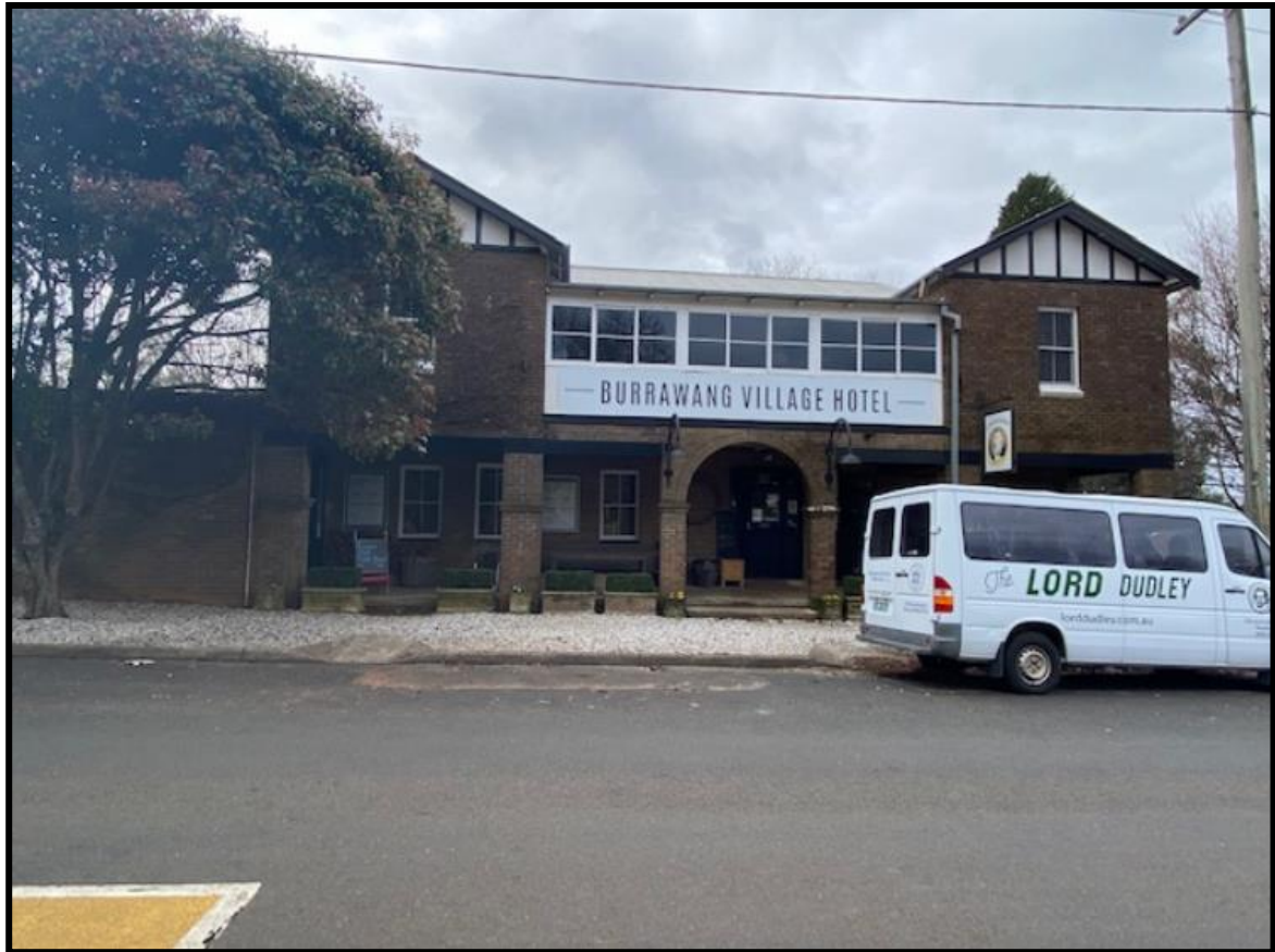
Figure 3: Street View Photo – No 14 Hoddle Street, Burrawang
