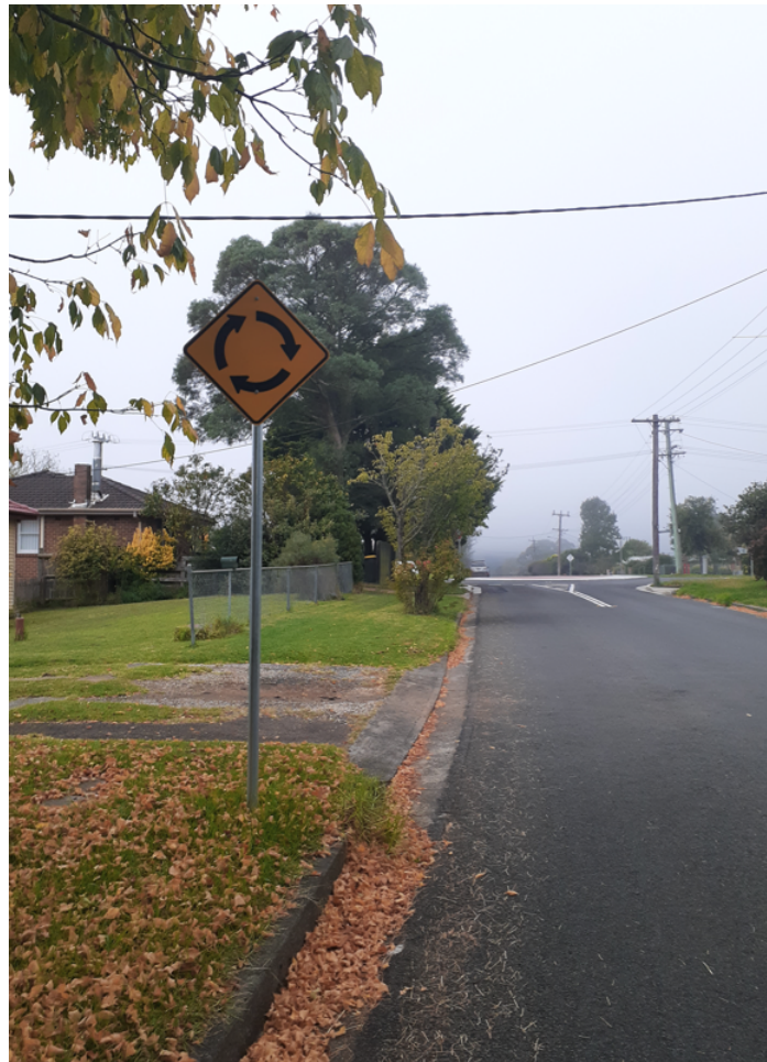
Image 5 - Existing W2-7 ROUNDABOUT AHAD sign on the western approach
