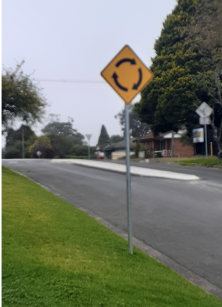
Image 1 - Existing W2-7 ROUNDABOUT AHAD sign on the northern approach
