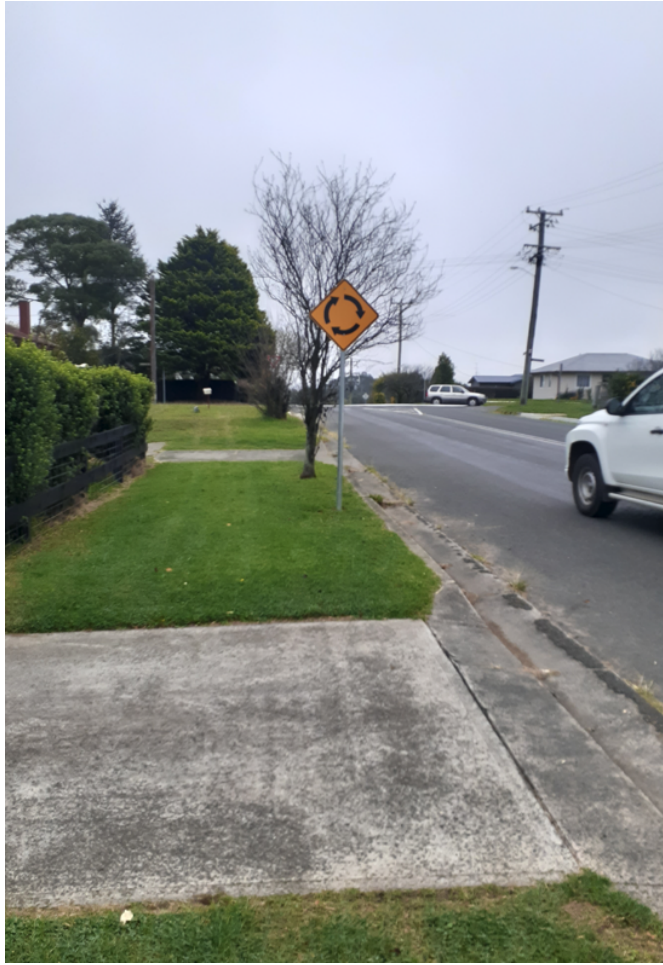
Image 3 - Existing W2-7 ROUNDABOUT AHAD sign on the southern approach
