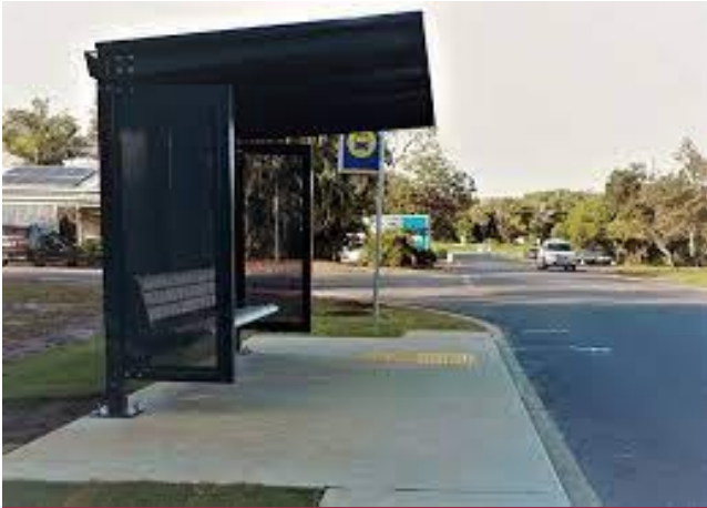
Country Passenger Infrastructure Transport Scheme Grant - $40,000
