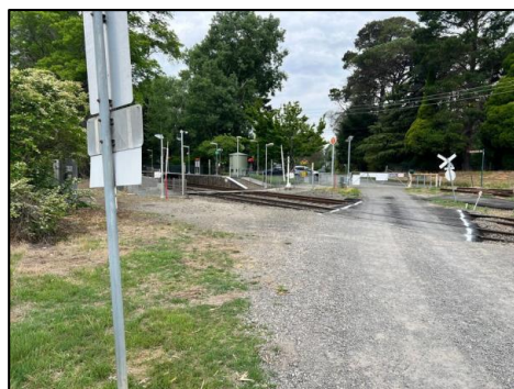
Security gated railway crossing that limits access
