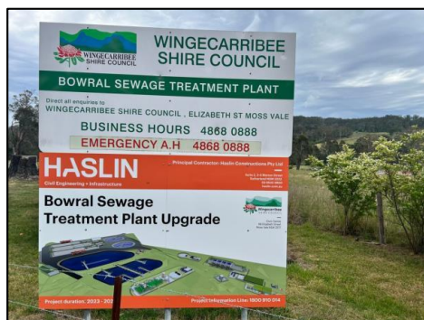
Adjoining Bowral Sewage Treatment Plant undergoing upgrade
