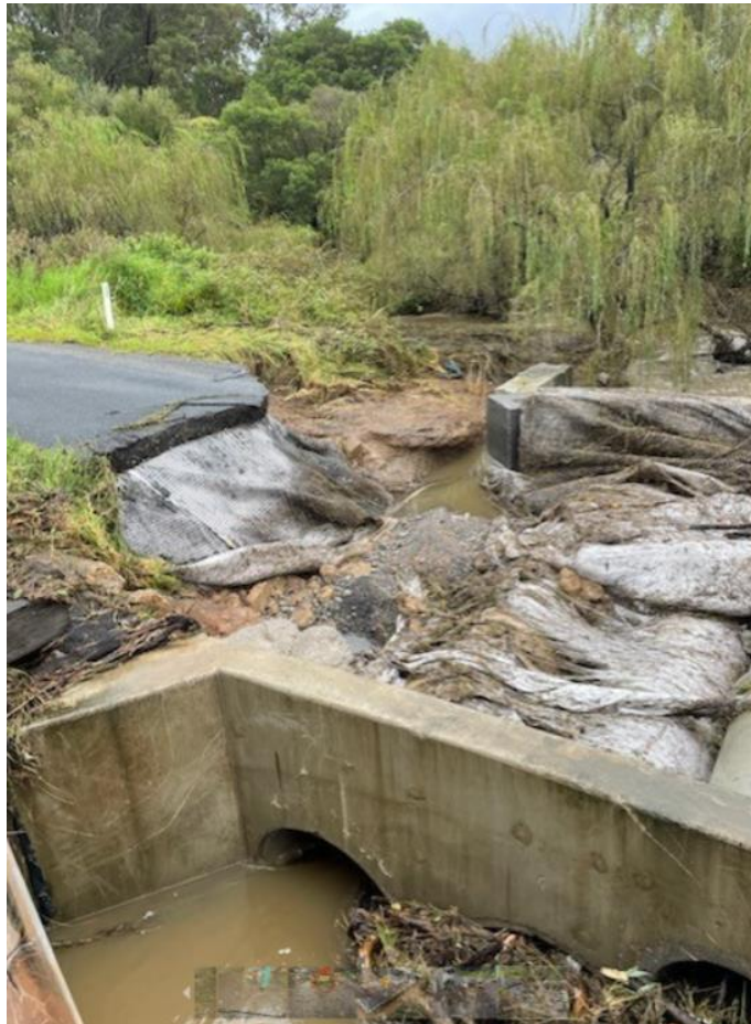
Photo 3.4.4—undersized culvert structures lead to a higher frequency of overtopping and pavement damage. The preferred and safer solution is to replace the culvert structure with a larger more resilient culvert solution less prone to blockage. Any new structure should be designed for partial blockage in major events with appropriate road, batter, inlet and outlet treatment. A cheaper, less desirable flood prone option is to replace the road pavement with a section of concrete causeway with appropriate upstream and downstream protections. This may reduce loss of the road infrastructure but leaves the road vulnerable to being cut in flood events, creating an impasse for emergency services and a higher risk to the community using the road.
