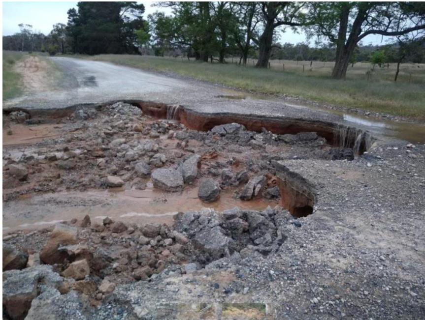
Photo 3.2.3 – Larbert Road, Braidwood. Road wash-out due to a lack of table drains and transverse drainage across the roadway (Common example courtesy of Queanbeyan Palerang Regional Council).
