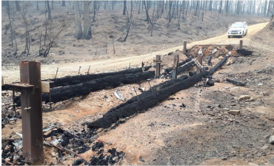
Photo 3.2.3 – Belimbla Bridge Eurobodalla Road was one of 18 timber bridges burnt in Eurobodalla during the 2019-20 bushfires severing access to the western agricultural, Forestry and National Parks area of Eurobodalla (courtesy of ESC).
