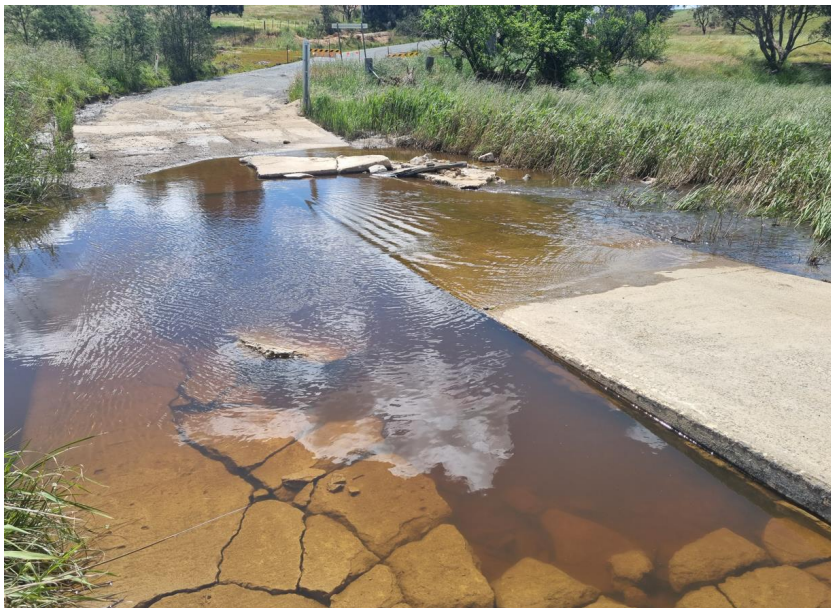
Photo 3.2.7 – typical causeway structure in very poor condition (photo courtesy of Upper Lachlan Shire Council). To build future resilience, structures like this one should be prioritized for replacement with a suitably sized bridge.
