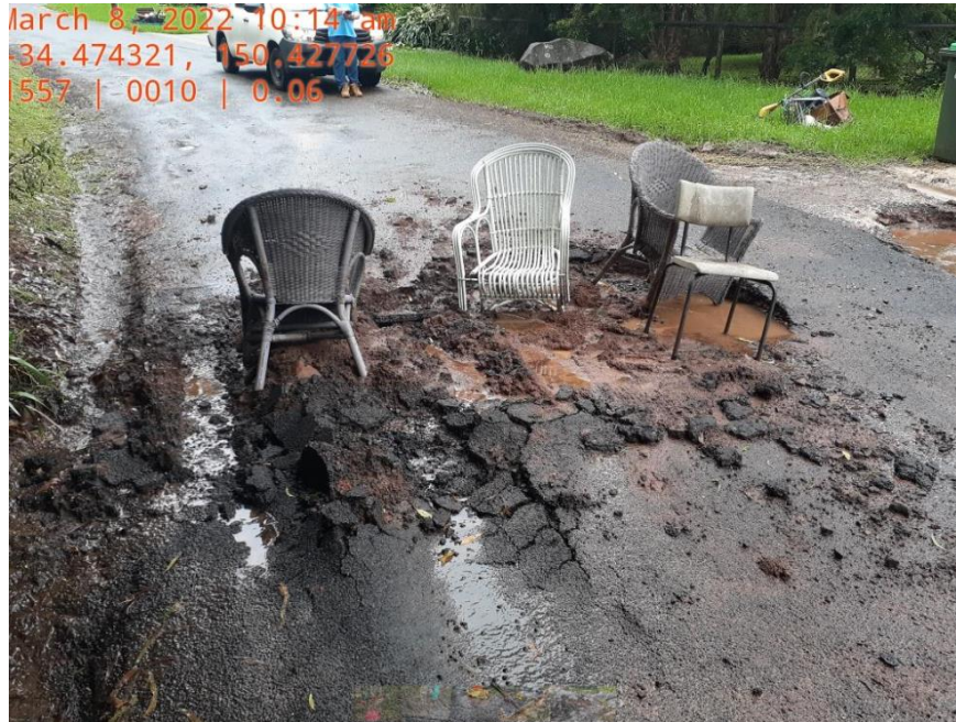
Photo 3.4.3 – sealed roads often hide road pavements constructed many years ago on poor wet sub-grades and/or poor-quality clayey pavement materials. When wet weather comes, the Council is often left with an expensive fix and adverse reputational impacts (courtesy of Wingecarribee Shire Council). Pavement testing can help Councils better understand the risks but is often beyond the affordability of Councils to undertake on a network wide basis.
