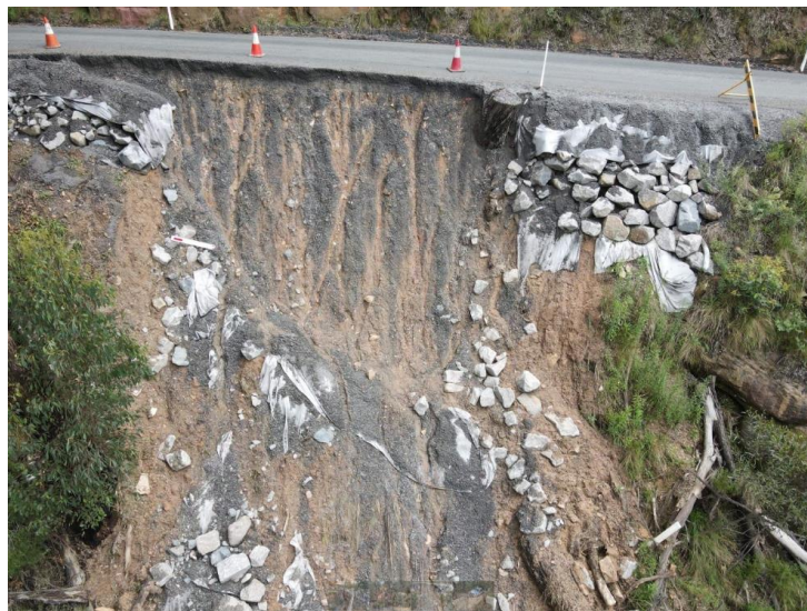
Photo 3.2.2 – Landslides are highly problematic to recover post disaster and require longer lead times, highly specialised geotechnical design, drill testing, tendering under the LG Act 1993 and delivery of
