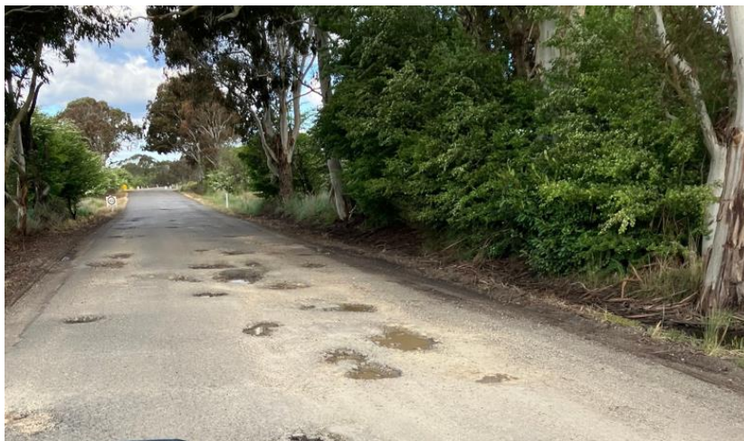
Photo 3.6.1 – typical example of a road with a very flat longitudinal grade and almost no road crossfall. The roadside vegetation is also constraining appropriate table drain clearing, shaping and maintenance. The inevitable result is that water is held on the roadway causing potholing and premature road failure. Filling the pothole is only treating the symptom, not the primary cause, resulting in repeat failures and a high level of community frustration (courtesy of Upper Lachlan Shire Council)
