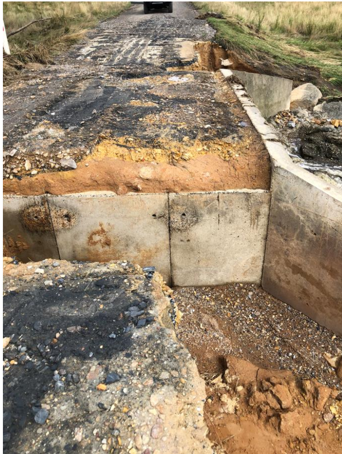
Photo 3.2.4 – typical undersized culvert structure with poor resilience when overtopped. Repairing this structure will leave this road vulnerable to repeat failure and damage. With specialist engineering knowledge, the capacity of this existing culvert can be improved at a moderate cost and/or the structure made more resilient to overtopping. Preferably though this structure would be replaced with a larger culvert structure and these existing box culverts re-used elsewhere on the local road, taking a more planned network wide approach. Regrettably, the inflexibility of the NDDRA means optimum solutions are often not able to be achieved (courtesy of Upper Lachlan Shire Council).
