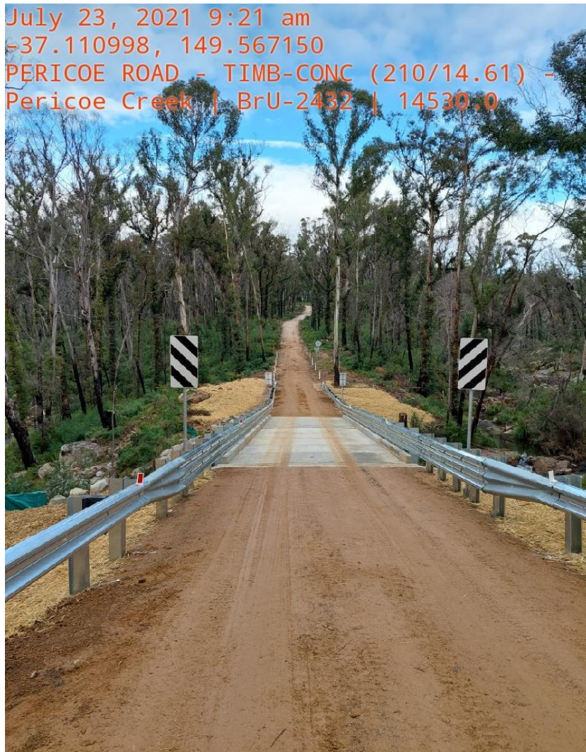
Photo 3.2.2 – Pericoe Bridge Pericoe Road, Towamba (courtesy of BVSC) replaced with a new bushfire resilient single lane concrete bridge
