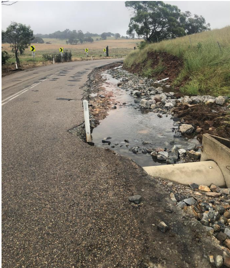
Photo 3.2.5 – Example of a legacy issue with an undersized culvert with the pipe inlet installed too high, resulting in high stormwater flows running along the road table drain rather than safely under the road through the culvert. The outcome is eroded table drains and excessive water saturating the downstream road pavement, causing a loss of pavement width on a tight curve and potholes in the ageing bitumen seal. Rectifying the road pavement without relaying and upgrading the culvert will inevitably result in future failures. Funding and specialist engineering advice is required to ensure issues like these are appropriately treated (courtesy of Upper Lachlan Shire Council).
