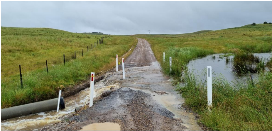
Photo 3.2.6 - typical under-sized culvert structure that is regularly overtopped causing repeat flood damage (courtesy of Upper Lachlan Shire Council). A new well designed larger culvert structure could be installed at relatively low cost to mitigate future damage, loss of farm access and future NDFA claims.
