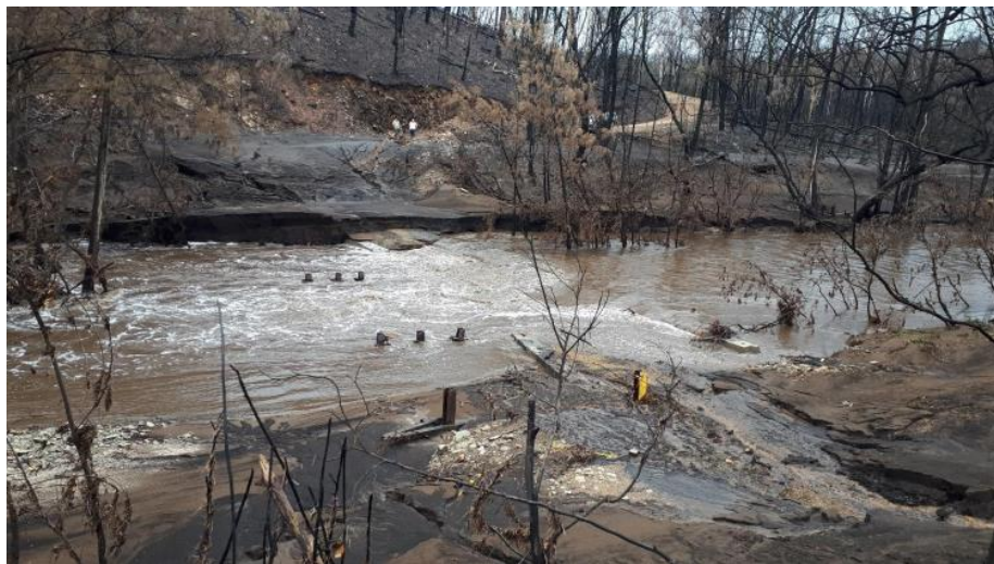
Photo 3.2.4 – Belimbla Bridge Eurobodalla Road (courtesy of ESC) Repeat flood disasters destroyed temporary access structures multiple times. Note the depth of ash debris on the banks of Belimba Creek.
