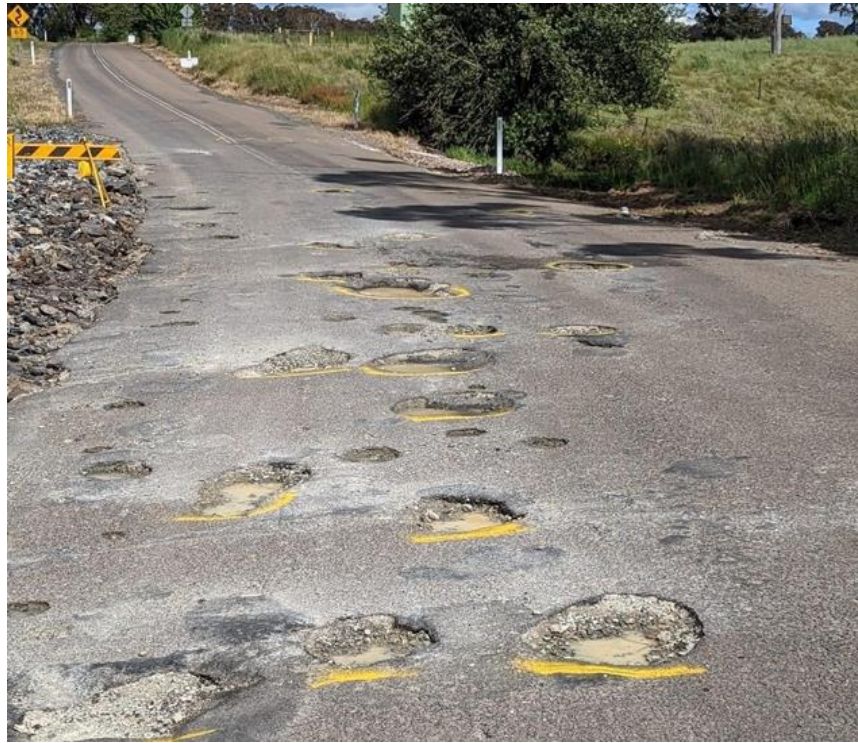
Photo 3.4.1 – local sealed road failing due to a combination of no batter catch drains and inadequate routine maintenance of table drains resulting in stormwater regularly flowing along the road. Combined with an ageing bitumen seal and flattening grades, potholing under traffic is inevitable (courtesy of Upper Lachlan Shire Council)
