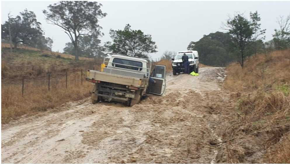
Photo 3.4.2 – weak underlying subgrade materials combined with high moisture levels require sound engineering methods to drain and strength the road before new structural pavements is built (courtesy of Upper Lachlan Shire Council)
