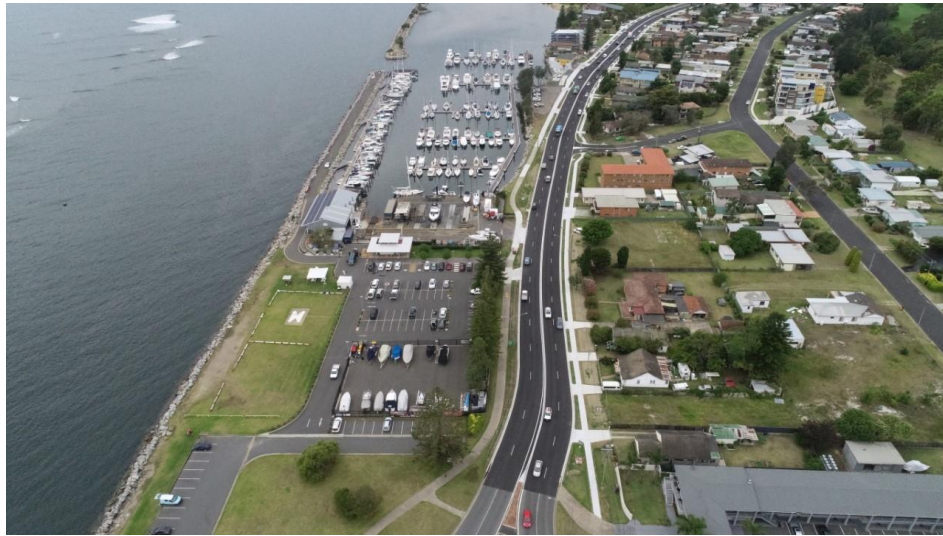
Photo 3.4.5 – Eurobodalla Shire Council lifted Beach Road Batemans Bay by about 300mm as part of this road safety upgrade. The road overlay was constructed as a highly resilient deep lift asphalt pavement with an associated drainage upgrade. The new pavement is more able to withstand the very high traffic loads (about 20,000 vehicles per day) and the overlay construction methodology assisted in adapting to future sea level rise as well as providing a cheaper and less disruptive construction method. The solution also better matched future redevelopment requirements for the adjoining medium density residential properties. Other sections of Beach Road near Hanging Rock reserve were previously lifted by up to 600mm using a mix of gravel sub- base overlain with a resilient deep lift asphalt pavement with improved drainage systems. All upgrade works were only made possible through external NSW and Australian Government grant funding.
