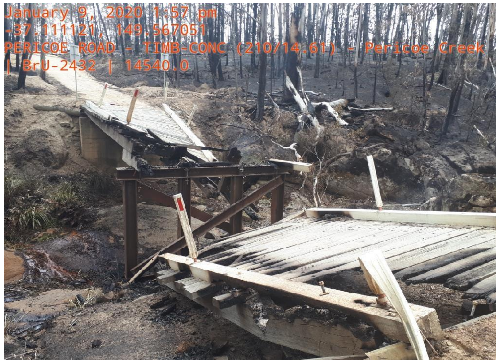
Photo 3.2.1 – Pericoe Bridge Pericoe Road, Towamba destroyed in the 2019-20 bushfires (courtesy of BVSC)
