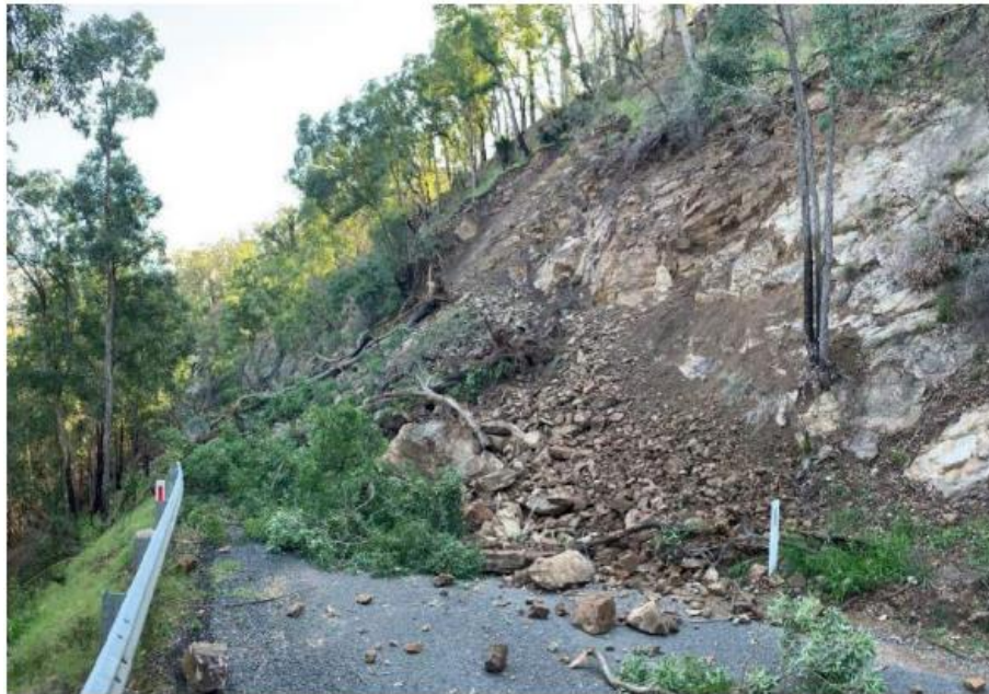
Photo 3.2.6 - Major 35m high landslide with an unstable embankment on Araluen Road Moruya West (courtesy of Eurobodalla Shire Council).
