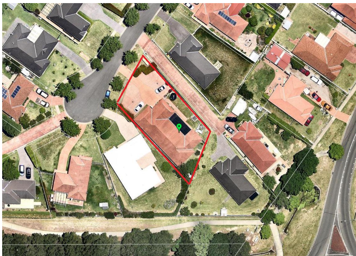
(Attachment 2 – Location Photographs) Figure 1: Aerial photo of site and surrounds - site outlined red (Source: Nearmaps)
