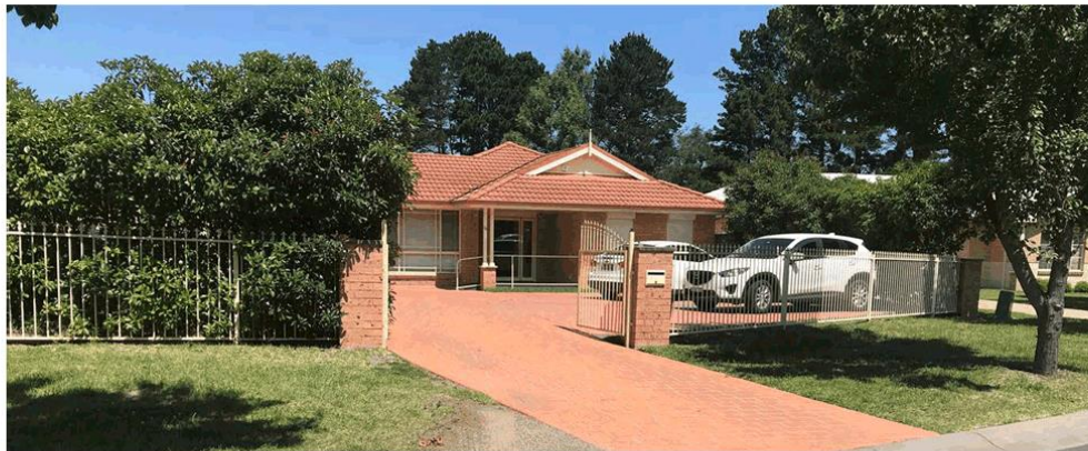
(Attachment 2) Figure 2: Site as viewed from the north west showing accessible entry porch and doorway
