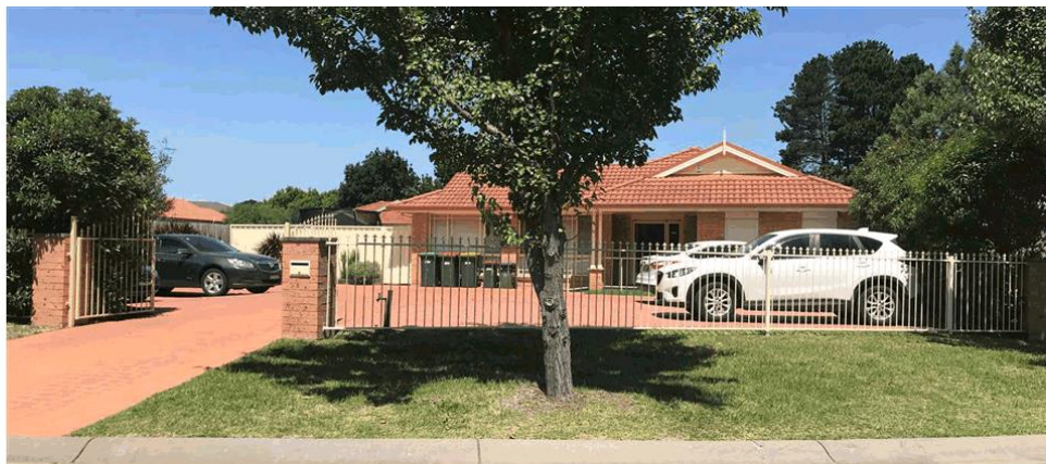
Figure 3: Site as viewed from the south west showing car parking and hard stand areas within the front setback
