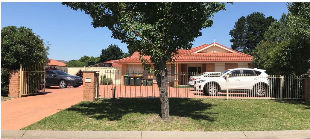
(Attachment 2) Figure 3: Site as viewed from the south west showing car parking and hard stand areas within the front setback
