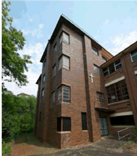
The main façade of the 1948 building showing its corner steel framed windows and four storey form. The building does not sit comfortably against the 1922 building.
