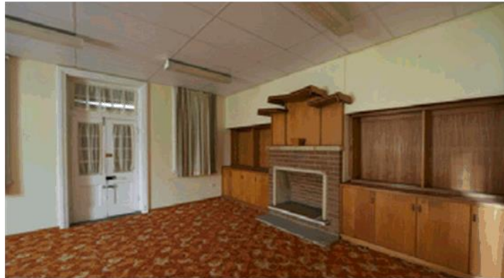
Interior of 1916 building, ground floor east end showing original French doors with 1968 joinery and grid ceiling fitout.
