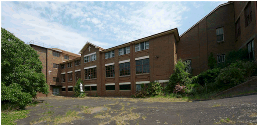
Main façade of west wing of the 1922 building, note the infilled verandahs and the removed castellated corner that is apparent in the earlier photos.
