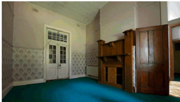
Interior of 1916 building, ground floor centre room showing original French doors with original fire surround, doors and pressed metal ceiling. This is one of two rooms to remain in the building without major change.
