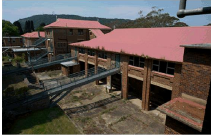
The rear elevation of the 1922 building showing its two and three storey form, note the excavation into the rear bank and the later steel bridges providing egress.
