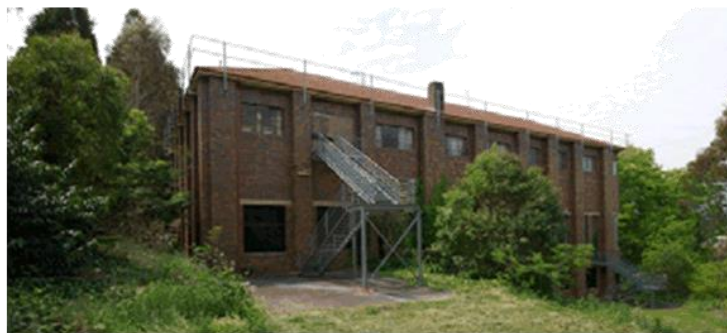
The rather undistinguished west elevation. It now features steel fire escapes and roof protection. The sloped nature of the site can be seen with the building stepping down having an additional lower storey to the south.
