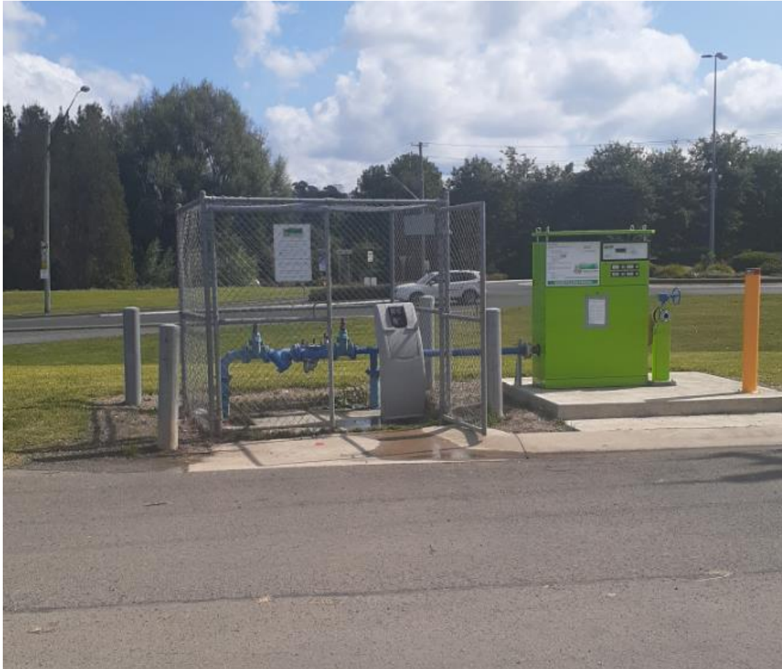
Image 2 – Existing Water Filling Station
