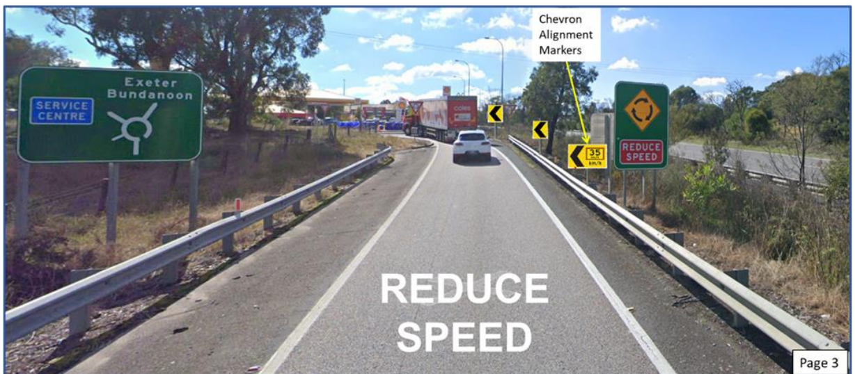
Fig. 3: Showing installation of additional Chevron Alignment Markers, REDUCE SPEED pavement marking.
