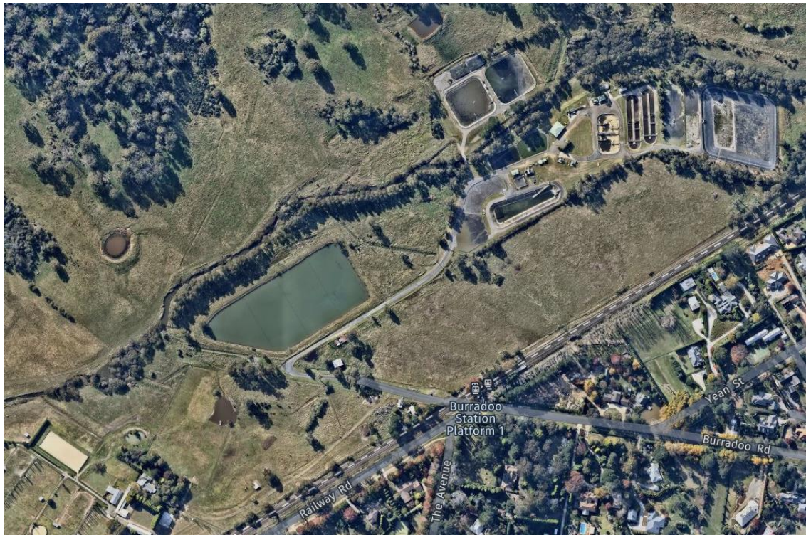
Image 1 – Aerial image showing Burradoo Road, rail level crossing and Bowral Sewerage Treatment Plant at the top of the image.
