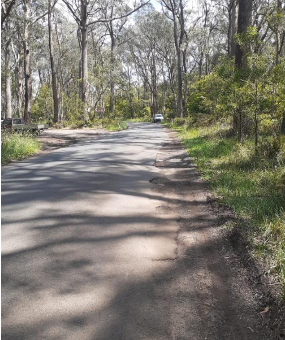
Image 2 – Existing narrow verge opposite the access to Bowral Lookout
