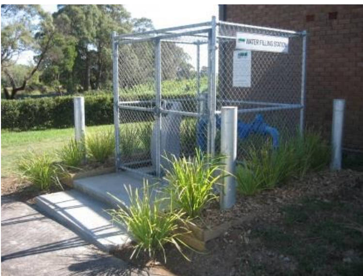
Moss Vale water filling station at Oldbury Road
