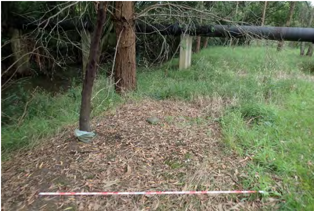
Plate 5: Existing pipeline in Activity Area, facing north-east.
