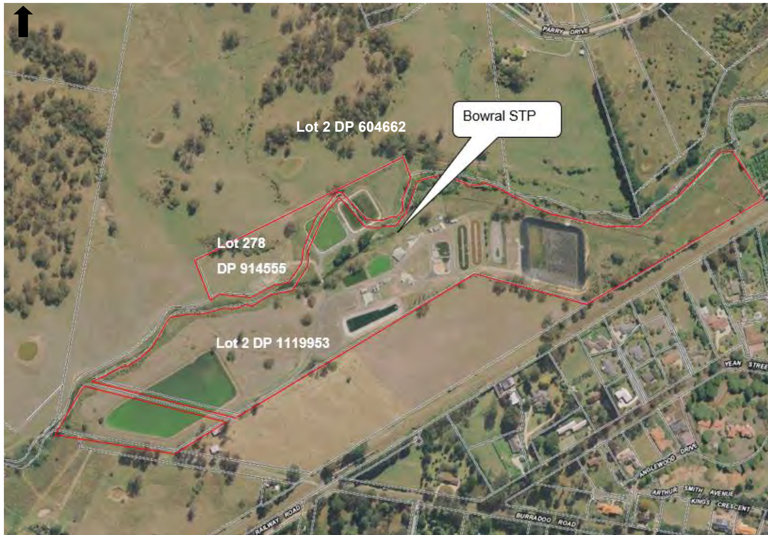
Figure 1-2 Aerial view of the existing Bowral STP site (outlined in red)
