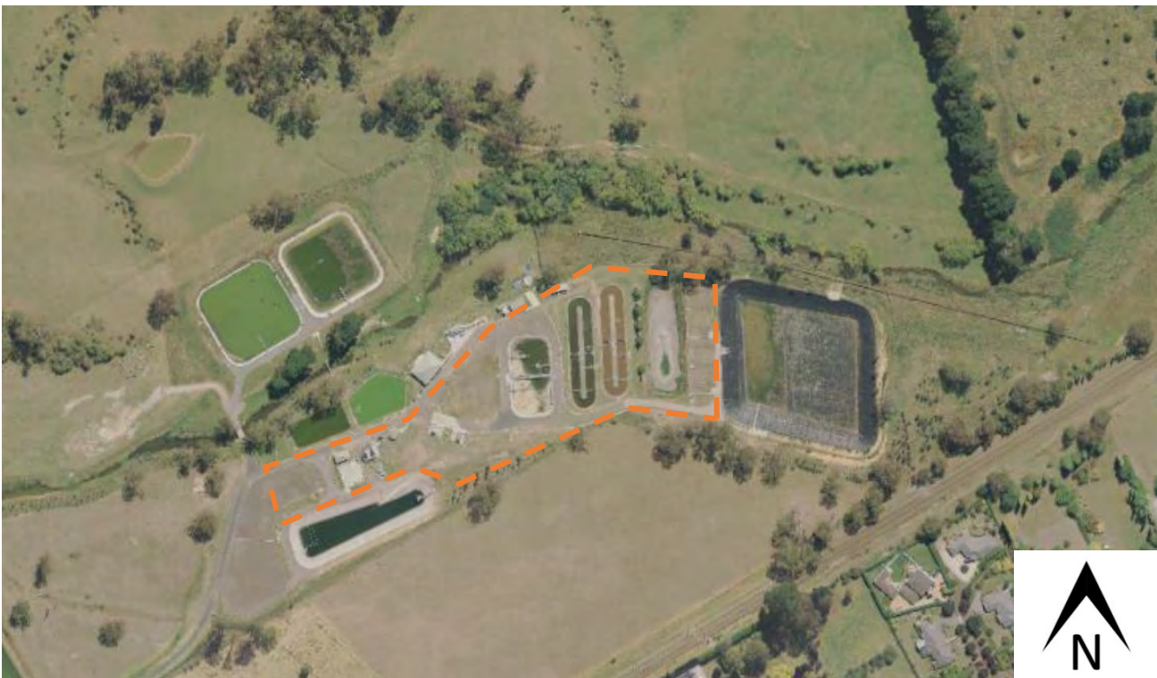
Plate 1 – Existing Bowral STP site layout/extents (Source: NSW Six Maps)
