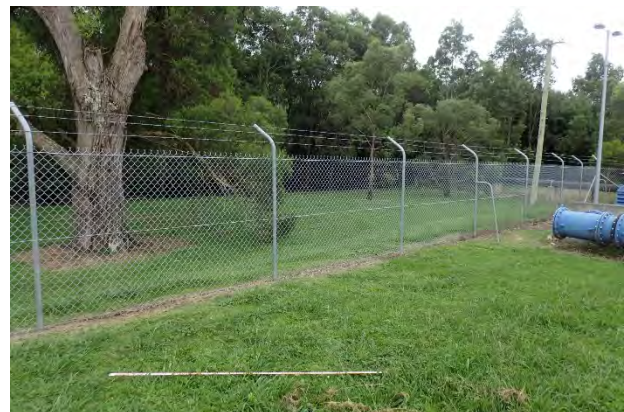
Plate 2: General location of revised pipeline facing north.
