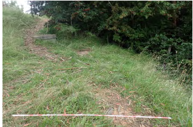
Plate 6: Location of ground surface connection of existing pipes, facing east.
