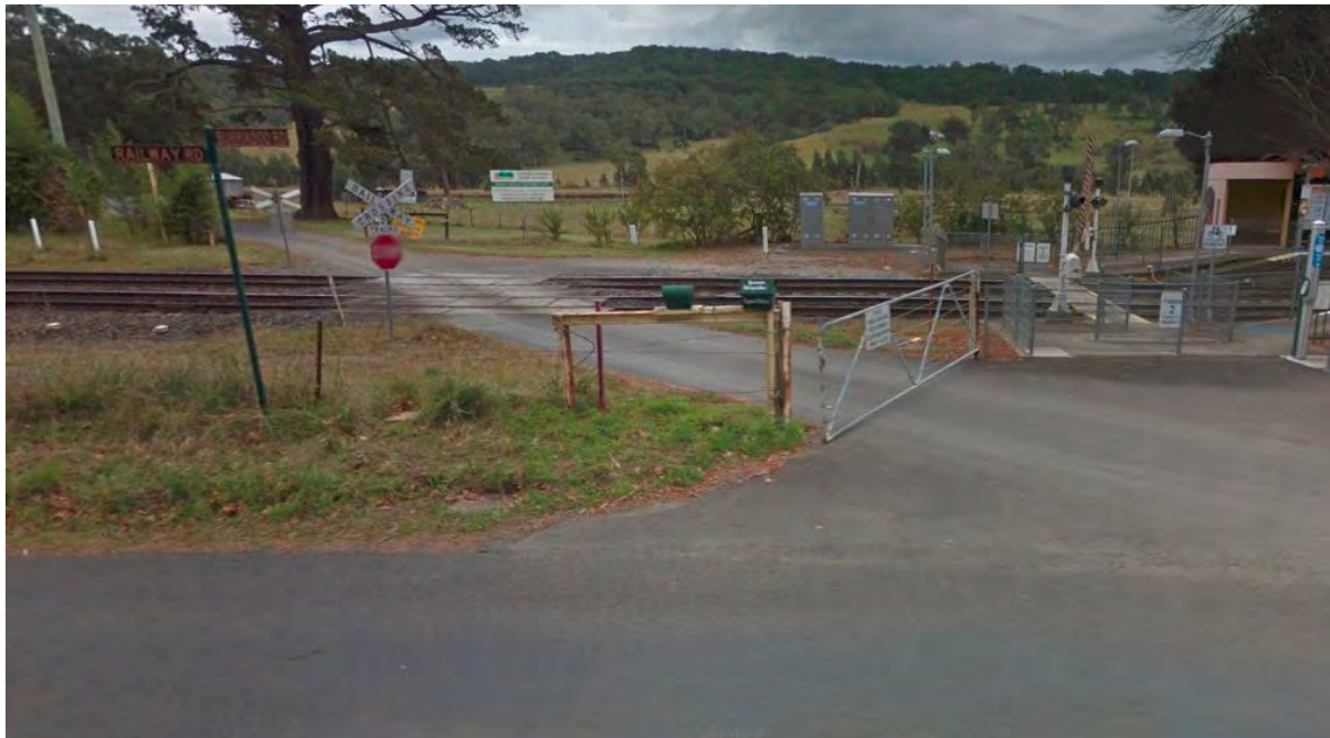
Figure 5-17 General Public view of Bowral STP from the Burradoo Road level crossing
