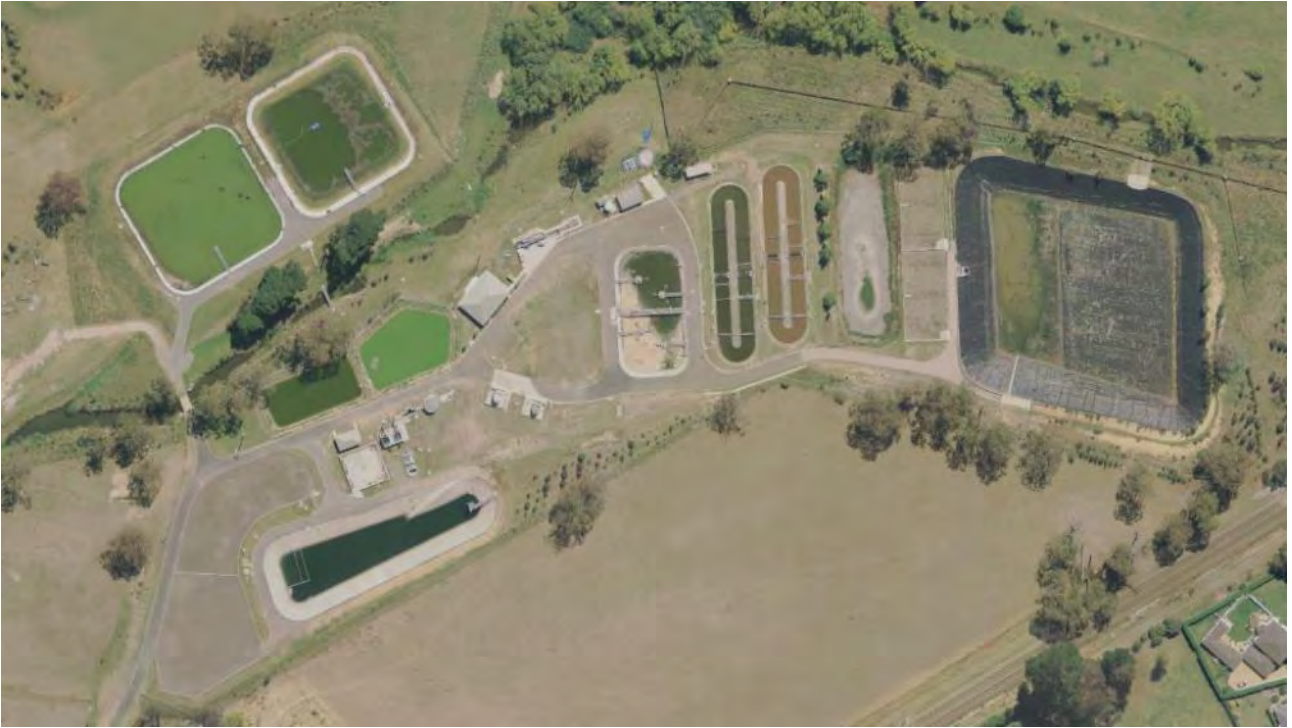
Figure 2-1 Aerial Photograph of Bowral STP
