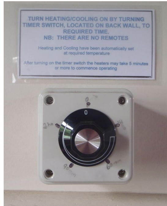
Figure 3: Control for air conditioner.
