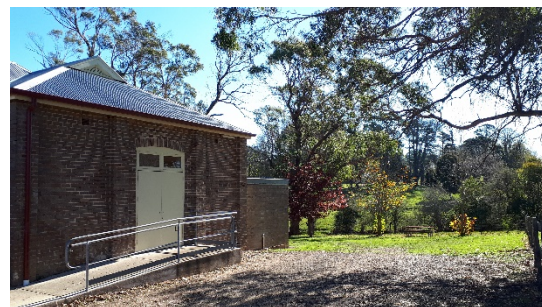
Ramp Access to Supper room
