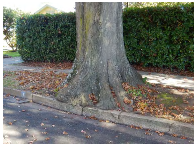
Figure 2.35 - Some interaction between trees and infrastructure is inevitable and needs to be accepted however the planting of large trees in narrow verges will create substantial maintenance issues and should be avoided. Holly Street, Bowral (Photo - Arterra)
