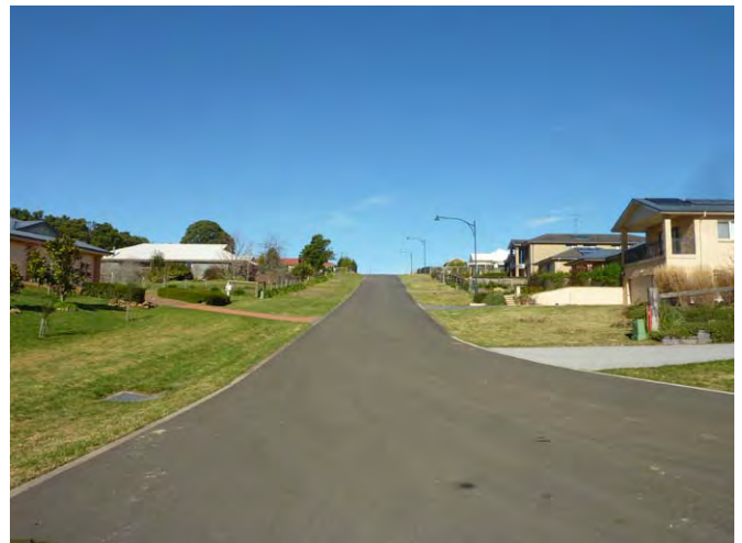
Figure 2.21 - Barrengarry Street, Robertson is an example of where larger street trees could be planted and grow without being compromised by above ground electrical wires. (Photo - Arterra)
