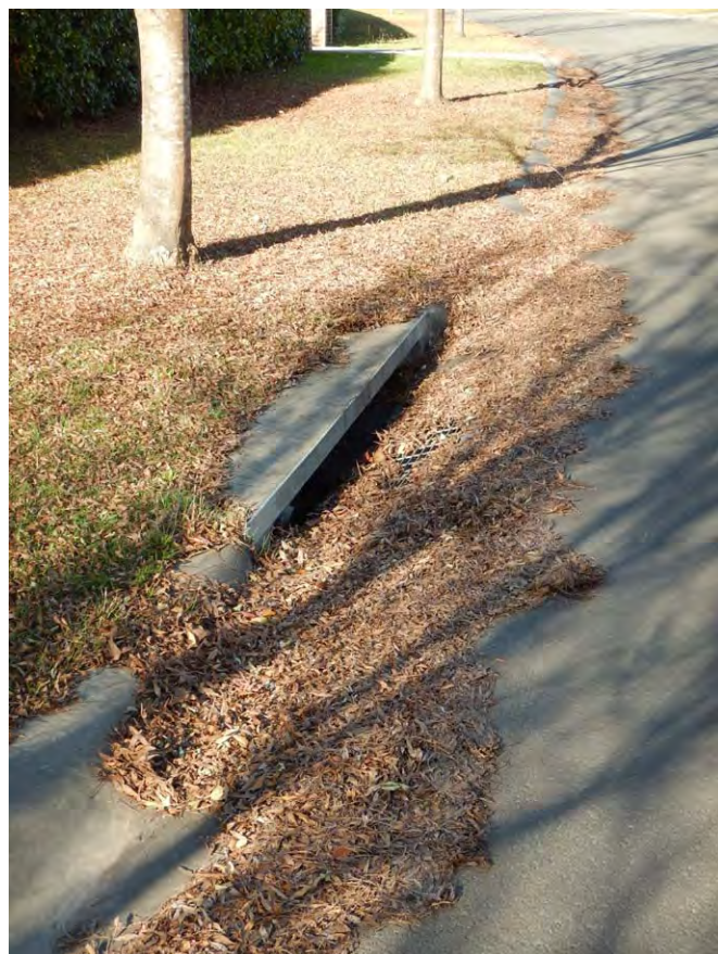
Figure 2.5 - Autumn leaf drop from Claret Ash on Highland Drive, East Bowral demonstrates the need for periodic cleanups to ensure drainage infrastructure remains functional. (Photo - Arterra)
