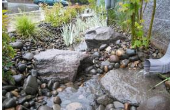
An example of a Rain Garden using recycled stormwater.
