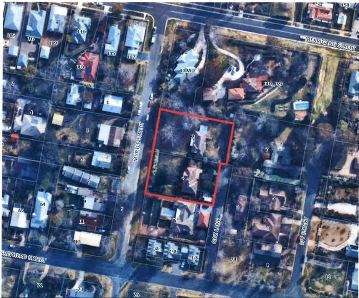
Figure 1: Aerial photo (17 August 2021) showing the housing mix in Myrtle Street and the substantial properties at nos. 2 & 4 (subject to IHO No. 12 and outlined in red) and neighbouring no. 6.
