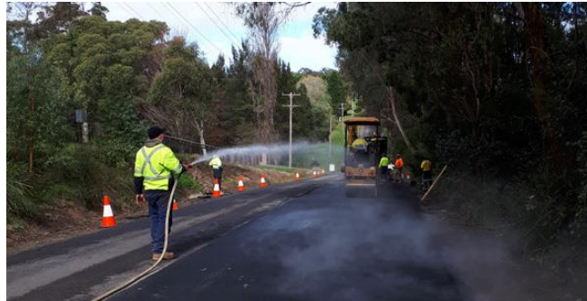
Priestley Street Culvert - Mittagong Robinson Street Culvert – Mittagong
