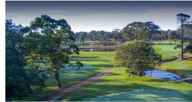
Construction of Bowral Golf Course Detention Basin 2022-2023 NSW Flood Recovery and Resilience Grant Program
