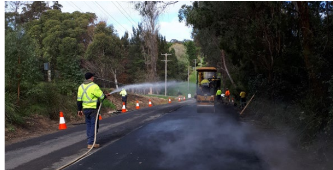
Berrima Road Deviation - New Construction Priestley Street Culvert - Mittagong Robinson Street Culvert - Mittagong
