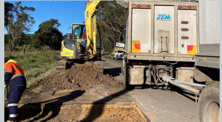
Old South Road rehabilitation project fast tracked
