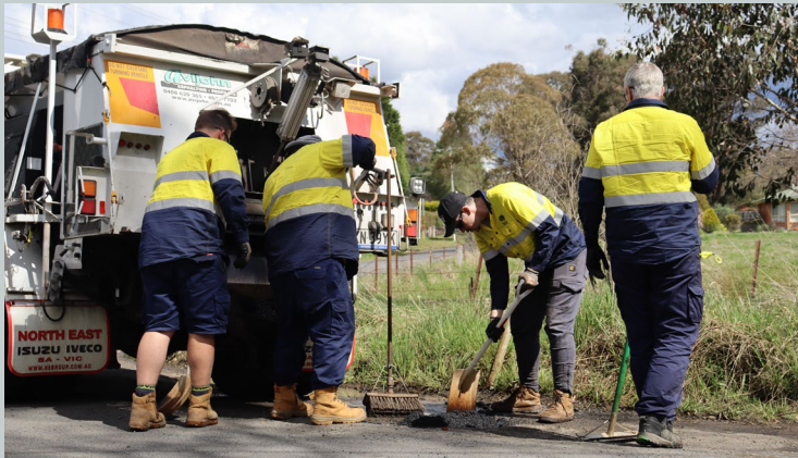
New pothole crew – 100 tones of pothole fill per week
