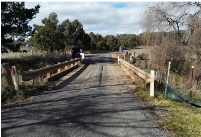
Ferguson Crescent Bridge Replacement Grant $2,899,000
