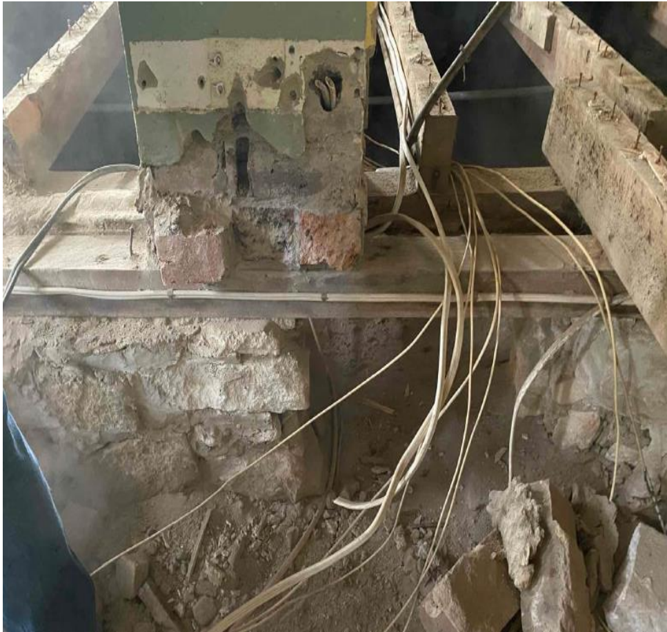
Failing footings in foyer floor
