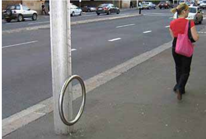
Figure 6.3 - Bicycle Parking Fitted to Existing Infrastructure
